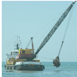
Dredging and Sediment Removal
