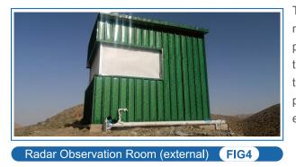
The HD-SAR300 is a rotating radar capable of 360° all-around monitoring. The rotating motion of the mechanical arm requires protective measures to prevent dust and moisture from affecting the instrument's accuracy and damaging the motor and transmission shaft. The design of the observation house not only protects the radar equipment, reduces maintenance costs, and extends the radar's service life.
