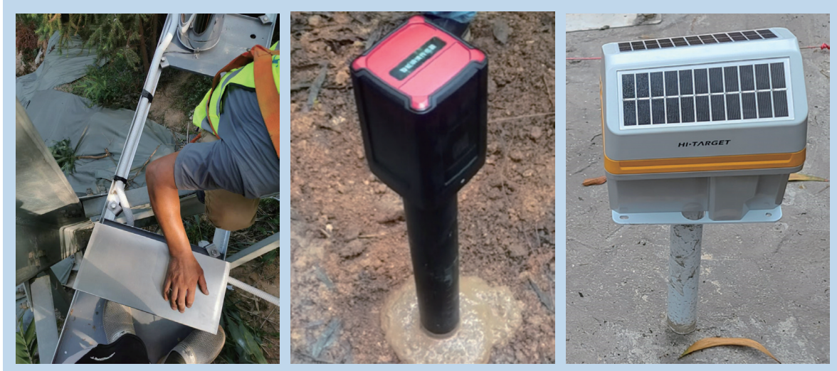
Soil moisture content meter GNSS receiver inclination accelerometer equipment installation FIG4
