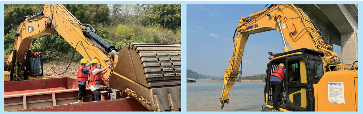
Equipment installation FIG3
