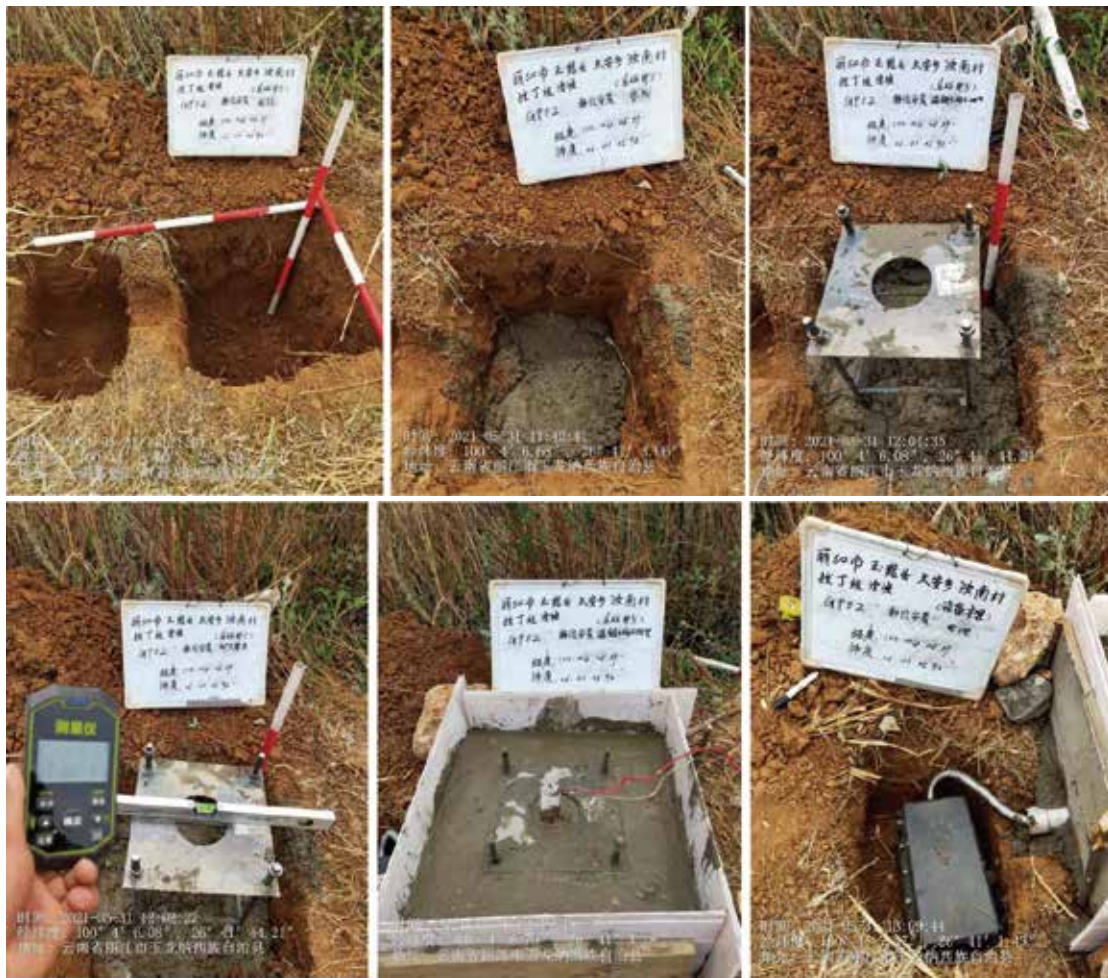
Foundation Construction FIG4
